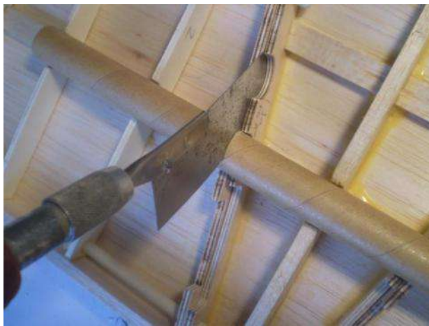
Cut the tube with a backless razor saw.
